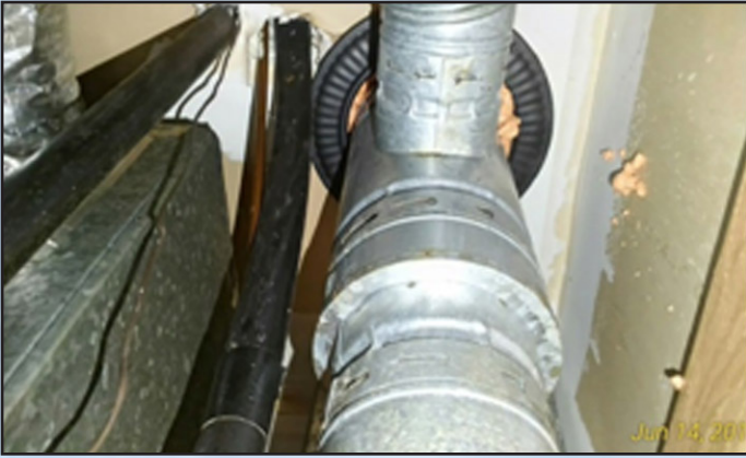
Sealing air ducts for better HVAC performance as an excellent weatherization measure
