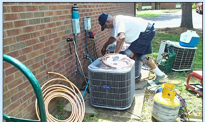
Contractor replacing HVAC condenser units that were emitting high levels of carbon monoxide
